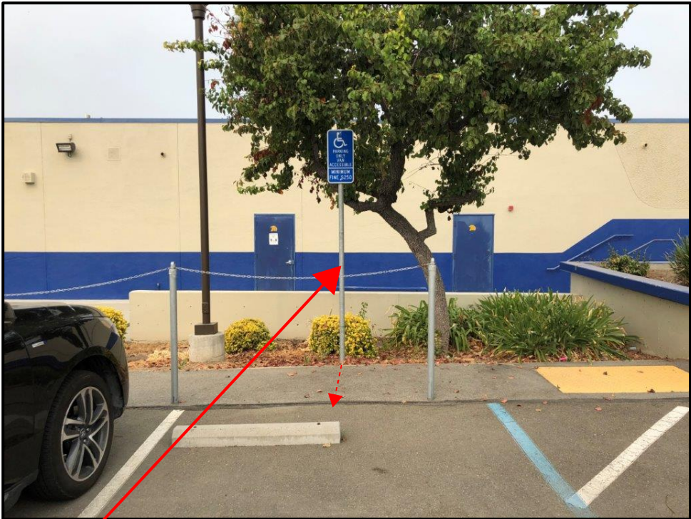
Photo 6: Relocate existing ADA parking sign and install new pole to be centered between new fence and wheel stop. Remove existing pole, footing, and backfill.
