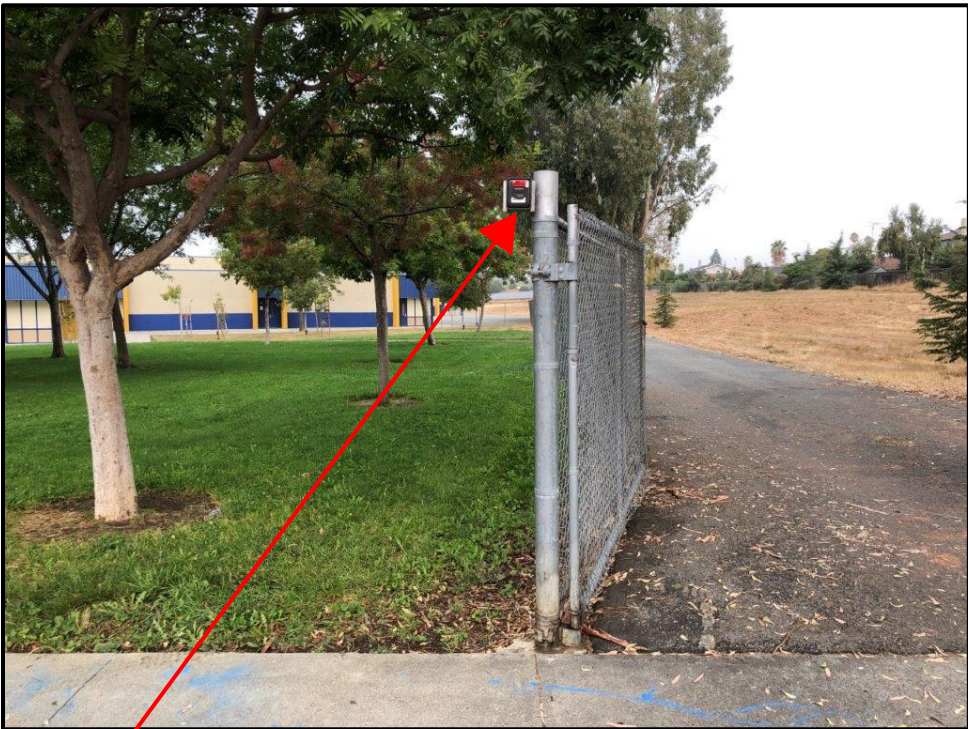
Photo 1: Temporarily remove knox box as necessary to accommodate for fence installation and reinstall at existing location.
